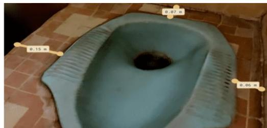
**Gambar 14. Dimensi Jarak Antara WC Jongkok Dengan Dinding Belakang & Dinding Samping**
