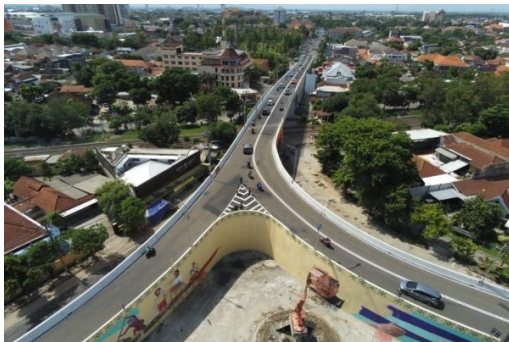
Gambar 8. Persimpangan Flyover Manahan (Sumber: Solopos, 2021)
