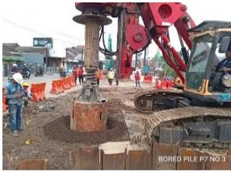
**Gambar 5. Crane Boring**
