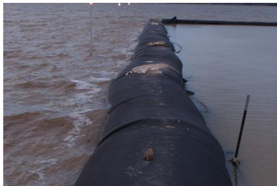
Fig.3 Geotube Breakwater
