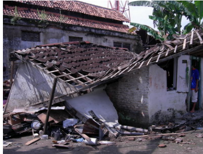
Fig. 1. Construction of a brick wall in residences that collapsed in the quake
