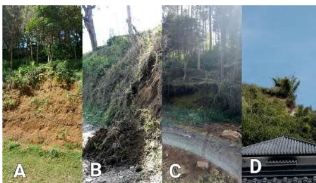
Figure 9. (A) Landslide around Ciwangun Indah Camp, (B) Landslide on the evacuation route of Ciwangun Indah Camp, (C) Old landslide in Ciwangun Indah Camp, (D) Landslides in Kampung Daun
