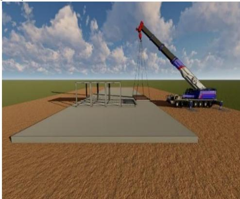
**Gambar 5. Erection Section Bottom Modular WG Flatpack**
