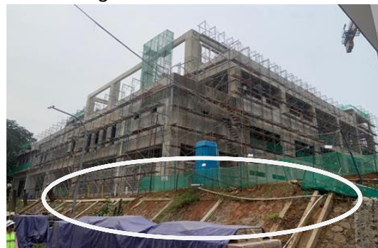
Gambar 11. Area ini belum memenuhi prinsip flexibility, safety and security.
