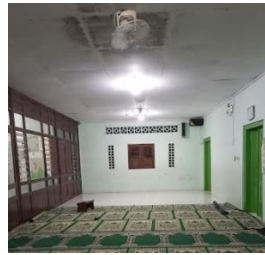
Gambar 12. Interior Selasar Kiri (sumber: Google, 2024)
