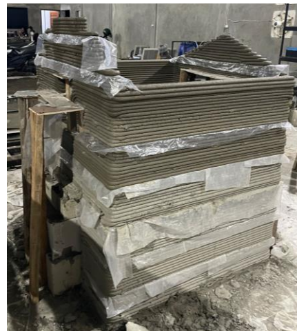
Gambar 5, 6 & 7. Proses 3D Printed berbasis mortar (sumber: Autoconz, 2025)
