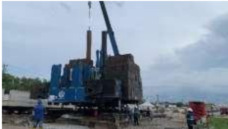
Gambar 6. Heavy Soil Pressure Digger (HSPD) (Sumber: Dokumen Pribadi, 2025)
