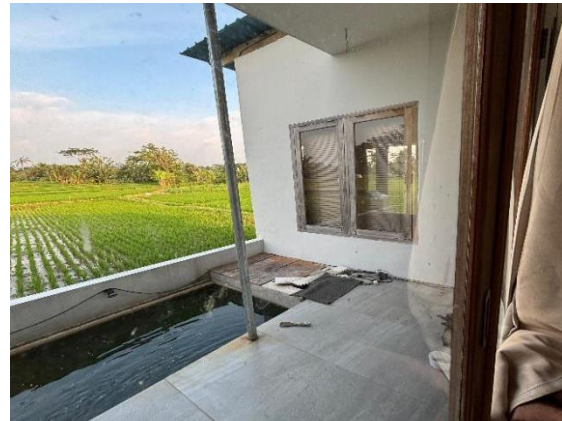
Gambar 3. Eksisting Teras Samping
