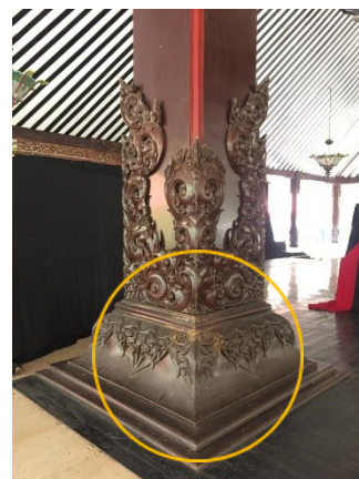
Gambar 7. Umpak Pendopo (Sumber: Survei, 2021)
