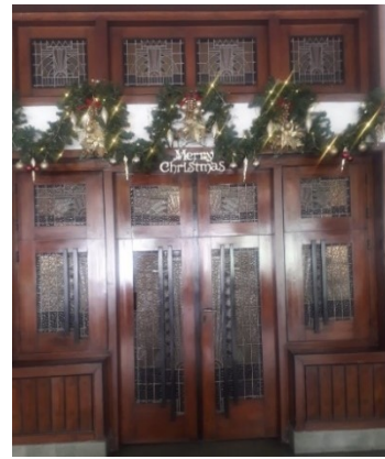
Gambar 15. Pintu Lobby Roemahkoe Heritage Hotel (Sumber: Survey, 2021)
