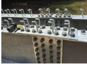
**Gambar 5. Sambungan Baut Girder**
