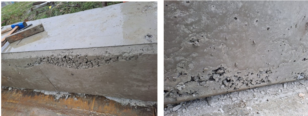
Gambar 5. Hasil capping beam bekisting baja
