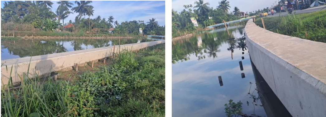
Gambar 4. Hasil capping beam bekisting kayu
